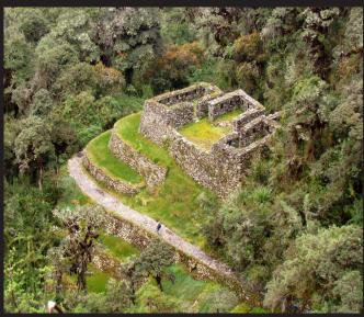
ture, which they managed to erect on the steepest slopes. The terrace wall structures were built up in a clever manner with best drainage systems to resist heavy rains and possible earth tremors. The filling consisted of various sized stones, pebbles, sand and fertile earth carried up from the river.
